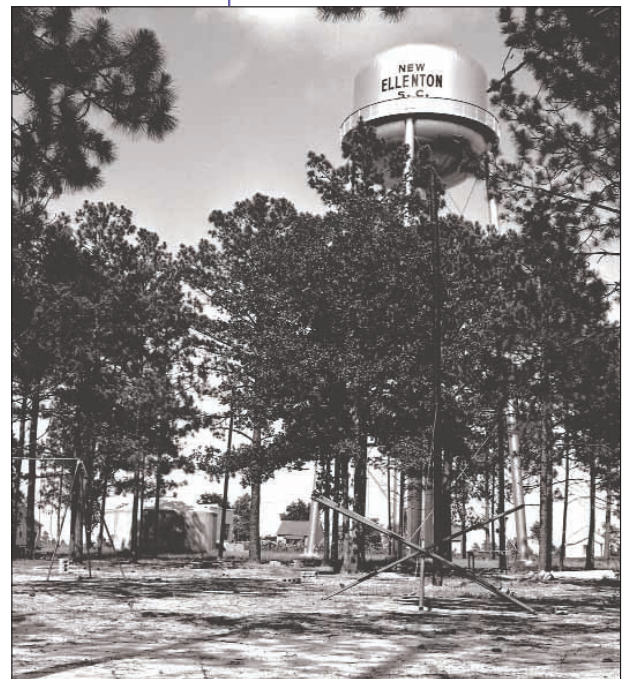
New Ellenton Water Tower and Buildings. Courtesy of SRS Archives, negative 2722-12.
