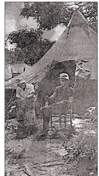
Some construction men lived in tents. This view showing two men, wearing hardhats, seated in front of a canvas tent appeared in a period banking magazine. Source: Burroughs Clearing House for Bank and Financial Officers , "Augusta, Georgia: The H-Bomb Brought a Boom," February 1952.
